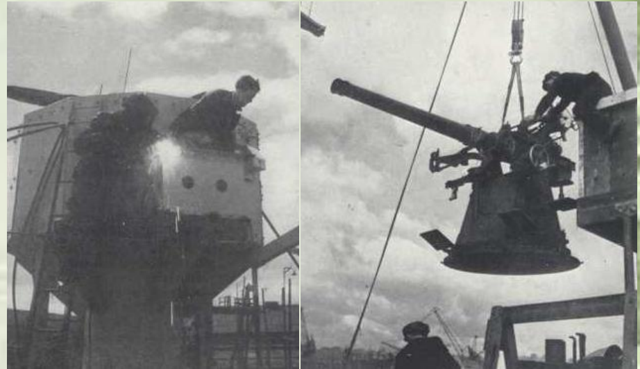
IN A LAST_MINUTE HUSTLE, while the new ship lies at the fitting-out wharf, guns are hoisted aboard, welders flicker over the gun platforms. She is almost ready.
