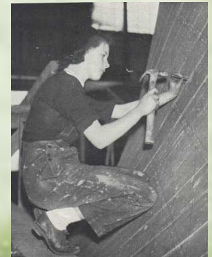
PATIENTLY knocking in rivets for the whole of a working day. She builds the wooden ships.
