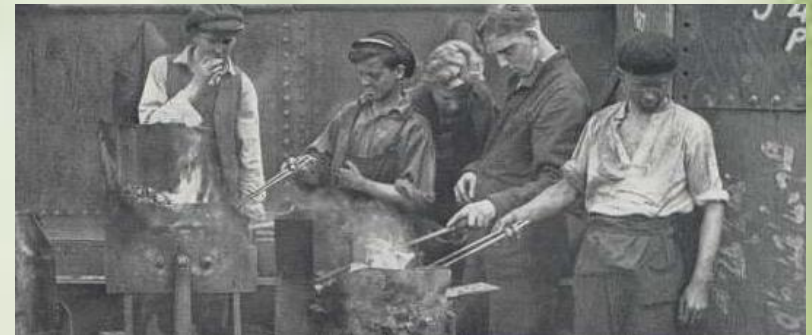
ON THE OTHER SIDE OF THE PLATE, inside the ship, are the heaters with their smoking braziers, plucking the rivets out of the fire.
