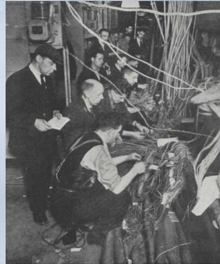
*Cables stripped of lead cover and insulation by fire.*
