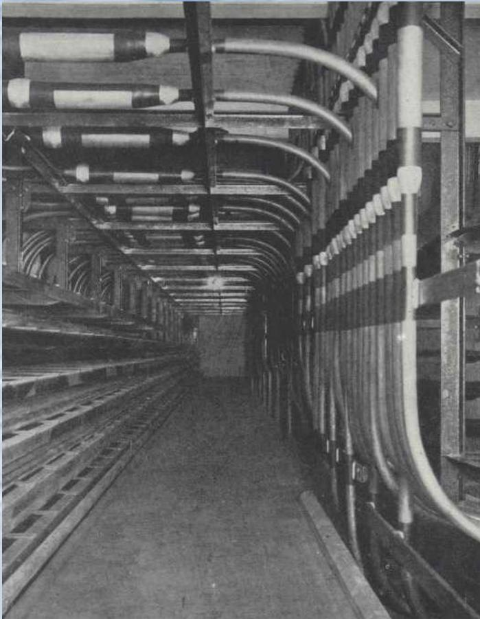
*Not Organ Pipes but Underground Cables serving a telephone Exchange.*
