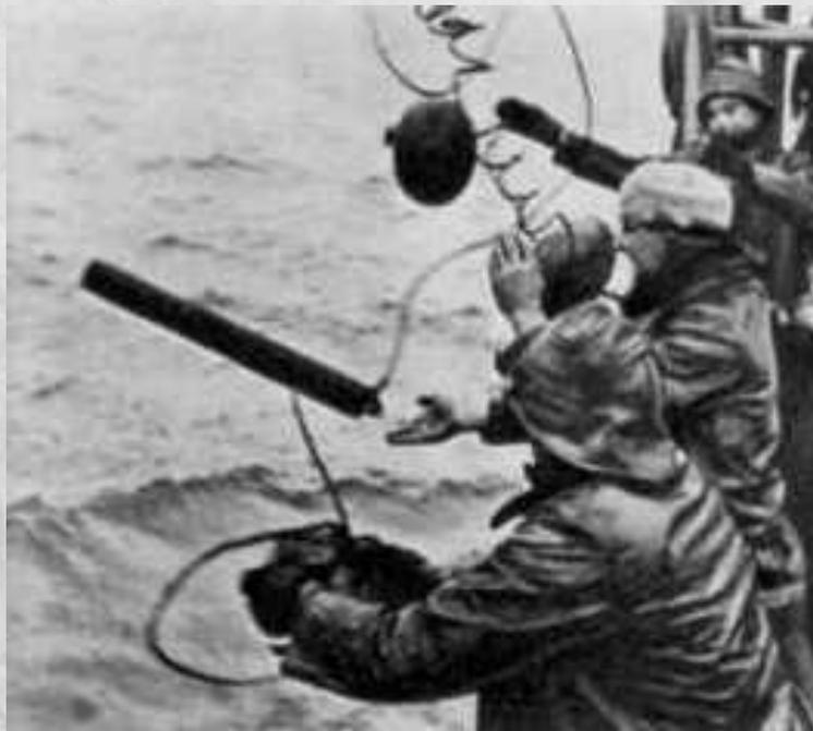
*THE "BOSUN'S NIGHTMARE", so called because of its tangles, was the first answer to the magnetic mine. The cylindrical bar is the sinker. Oval-shaped floats are called "blobs." The wire sweep is magnetized.*
