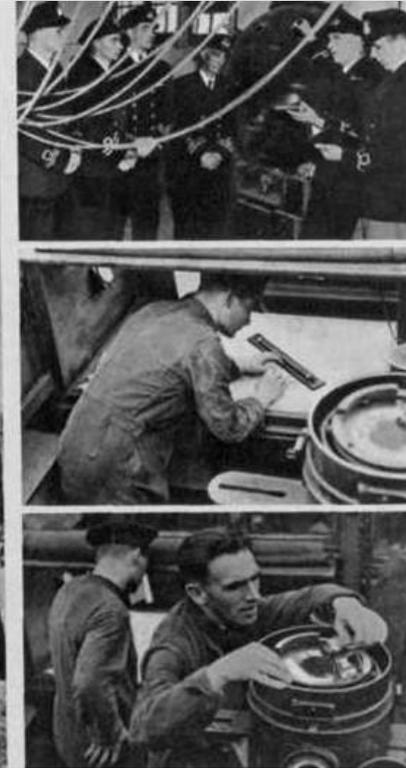
***THE MEN OF THE SWEEPERS.** Learn to be masters of their dangerous job in H.M.S. Lochinvar a shore establishment. Top left, rating trainees are taught wire splicing. Above; the mechanism of a mine is explained to officers, seen through the shrouds of a mine-dropping parachute; an officer studies pilotage; another takes a compass bearing.*
